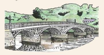
8 The Old Wye Bridge was the main road bridge into the town from Gloucestershire. It was built in 1816 and has been strengthened several times to accommodate increasing traffic volume and weight. The bridge is now a protected monument.
